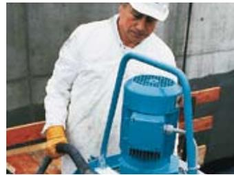
Slurry mortar guns (such as PUTZMEISTER Sprayboy with 8 mm nozzle) are suitable for the application of VANDEX BB 75 E.
