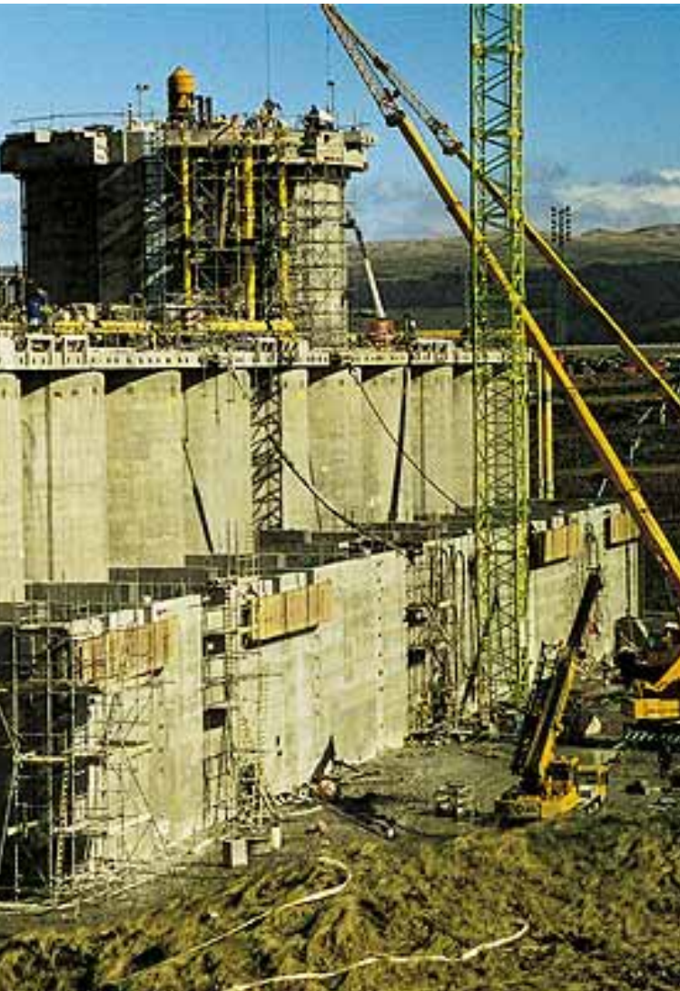
The oil rig base together with the crude oil tank weighing approximately 90,000 tonnes was towed using 4 tugs from its dry dock in Hunterston to the Harding Field in the North Sea.
