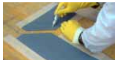
A Bond abutting tape ends (mitred, T-joints etc.) with instant VANDEX DILA JOINT TAPE ADHESIVE.
