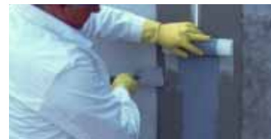
2 Place VANDEX DILA JOINT TAPE, followed by working fabric edges on both sides into waterproofing slurry.
