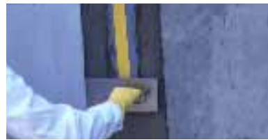
3 Embed fabric edges in second coat of VANDEX BB 75 E (3 kg/m 2 , 1.5 mm) and smooth surface with wet brush.
