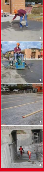
VANDEX SUPER dry-sprinkled as **powder** immediately after initial setting of concrete.
