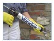
**4.** Back fill the hole fully with VANDEX IC to within 10 mm of the surface. Close the holes with VANDEX UNI MORTAR 1.
